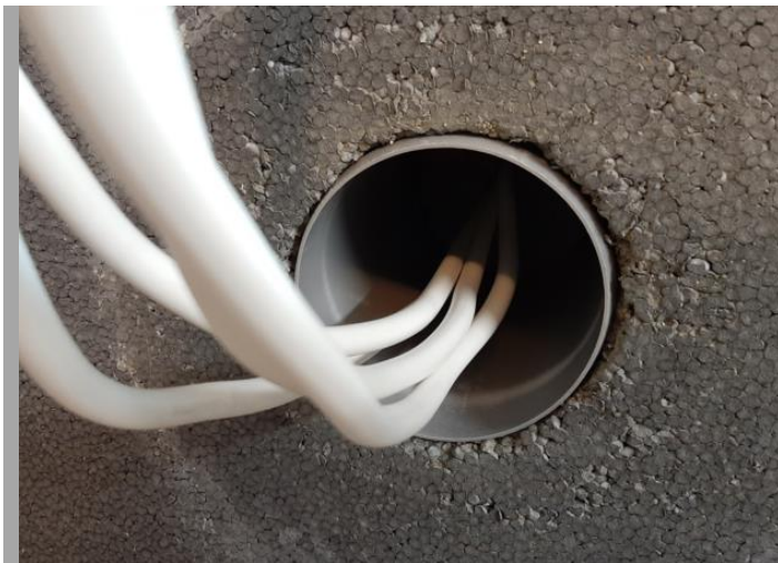
STEP 3: CLEAN THE DUCT FROM SOLID DIRT, DUST AND GREASE.
