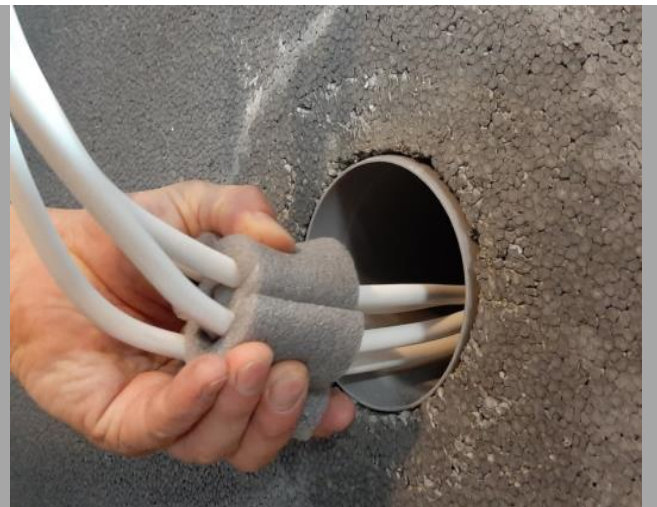
STEP 4: USE A FOAM OR PUR 2K FOAM (5 ÷ 7 CM LENGTH) AS SUITABLE BACKSIDE BARRIER AND TO SEPERATE THE CABLES FROM EACHOTHER.
