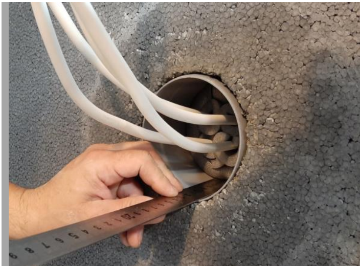
STEP 7: THE COMPOUND ANTICOR SEAL 511 SHOULD BY APPLIED OVER A LENGTH OF 10 ÷ 12 CM.
