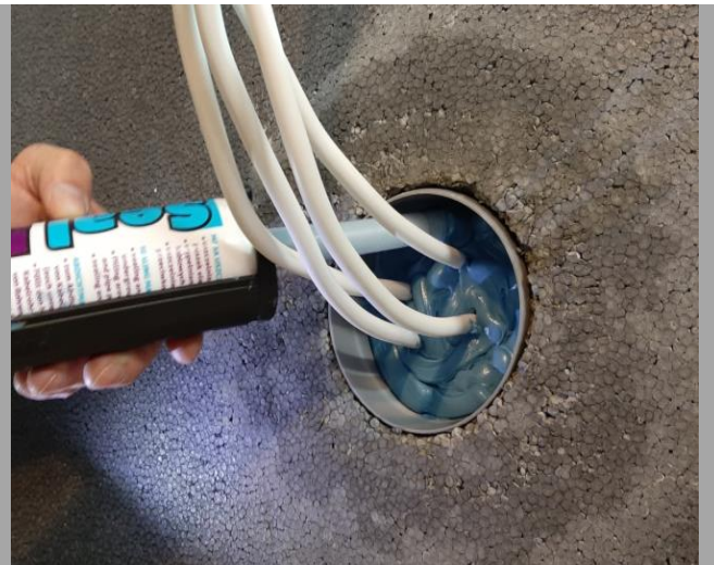
STEP 8: START INJECTION OF THE COMPOUND ANTICOR SEAL 511 WITH THE APPLICATION GUN AROUND THE CABLES. MOVE THE NOZZLE FROM SIDE TO SIDE, WHILE SLOWLY MOVING THE NOZZLE OUTWARDS.
