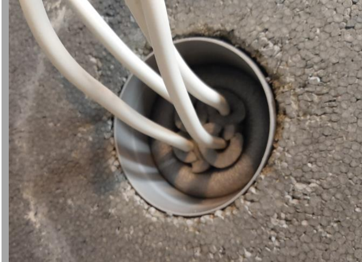
STEP 5: THE INLET IS PREPARED FOR THE NEXT STEP.
