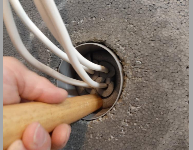
STEP 6: INSERT THIS BACKSIDE BARRIER AT THE DEPTH OF APPROX. 15 CM IN THE INLET.
